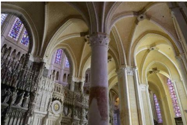
Above, top: Chartres Cathedral, with repainted vaulting in the choir contrasting with the existing nave and transepts in the foreground, Chartres, France, July 11, 2012
