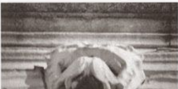
Heavy erosion forming hole in cornice
