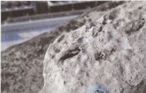
Heavy erosion forming hole in cornice
